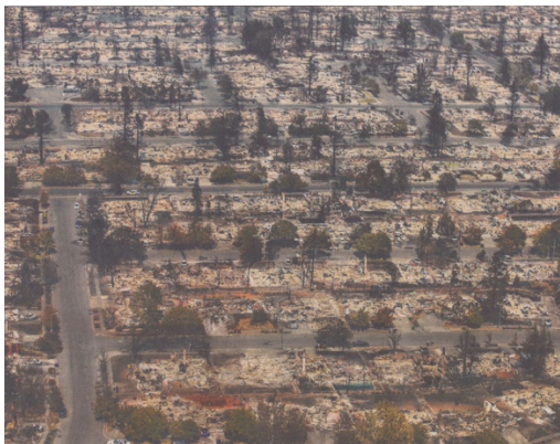
Trees remained in Coffey Park, Santa Rosa, while all structures were lost.
