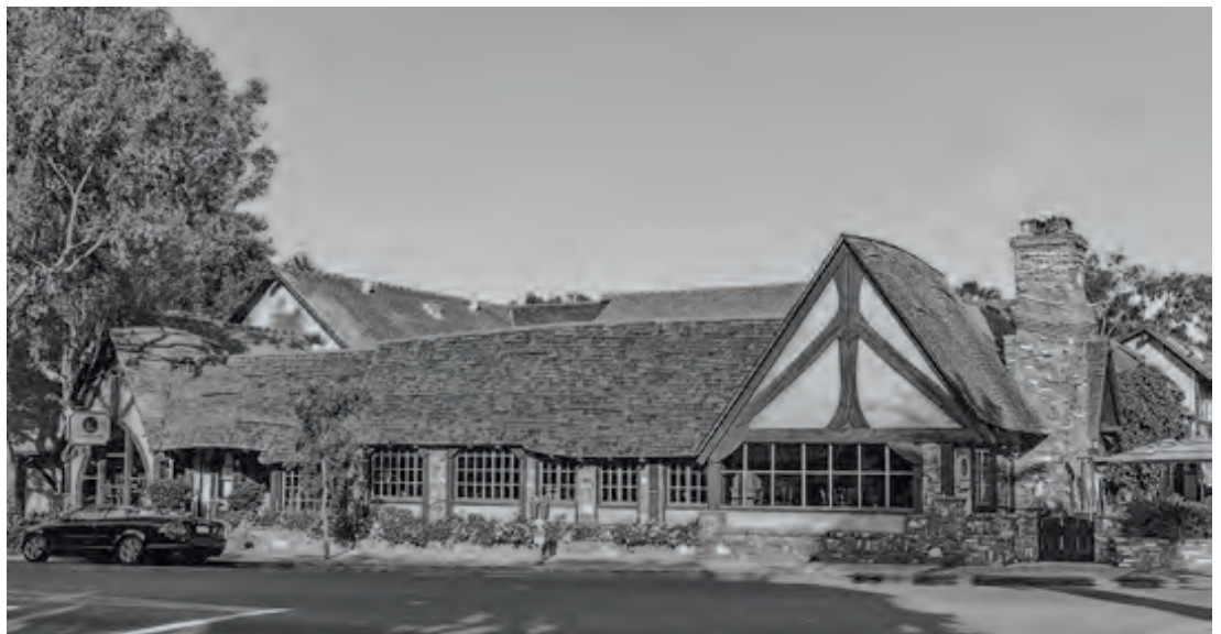
Lumberyard Building, Forest Avenue (Thomas A Lamb) 2016
