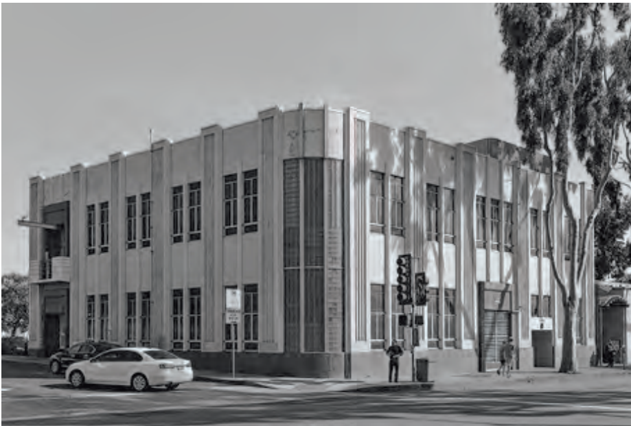
Verizon Building, Broadway and Beach (Thomas A Lamb) 2016
