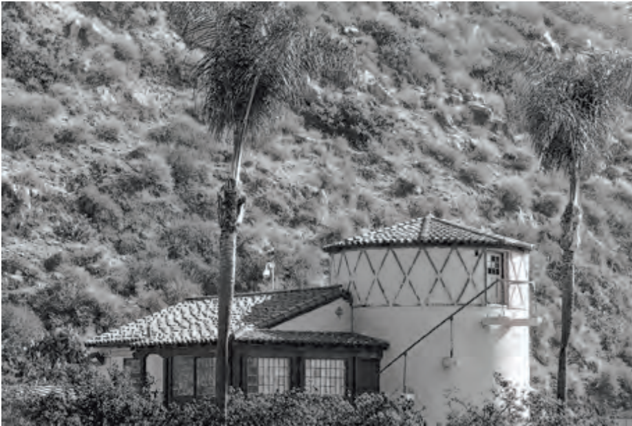
Sewer Building, Laguna Canyon Road (Thomas A Lamb) 2016
