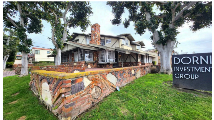
Chris Abel’s “interpretation of Tudor Revival” saved from transformation. They were even going to remove the chimney.
