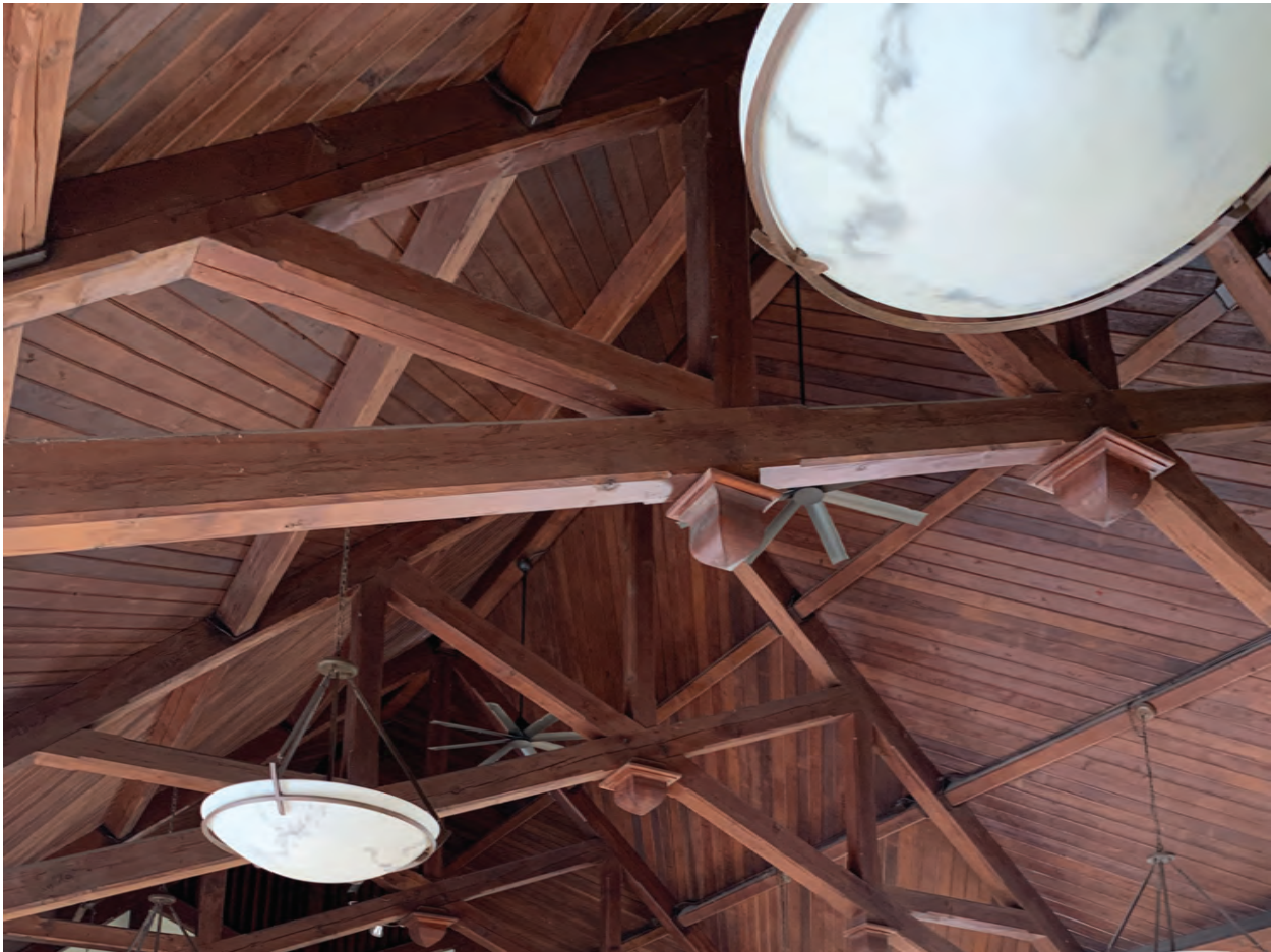
Truss detail of Bridge Hall ceiling, Hunter Fuentes photo
