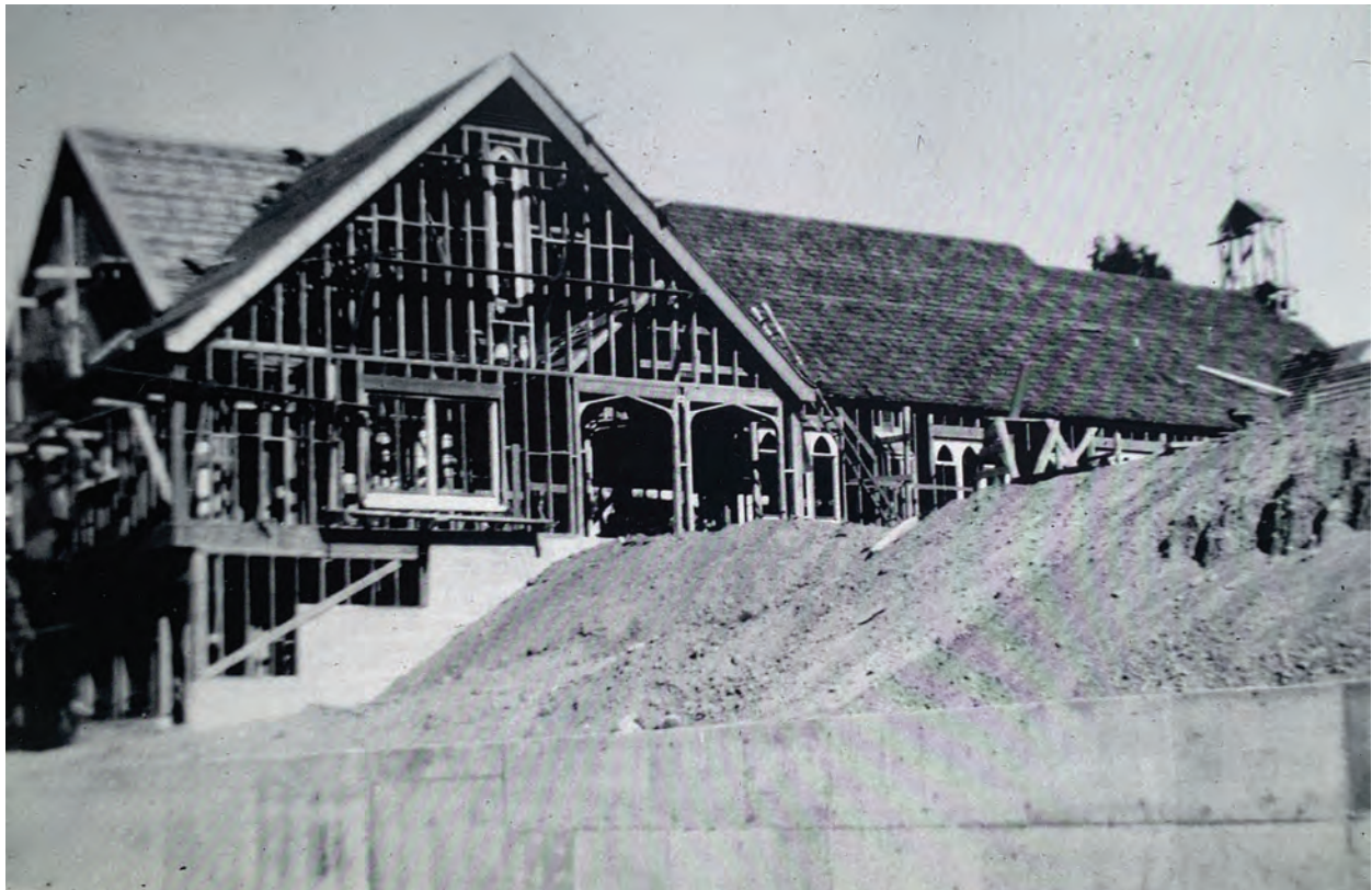
Bridge Hall under construction circa 1949
