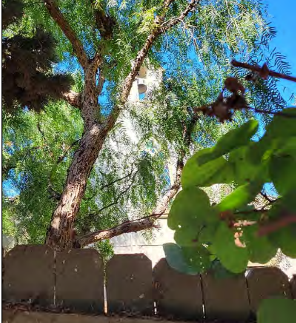
Photograph 2: Parish Hall, view northwest from subject property front yard. Bell tower is obscured by mature trees.
