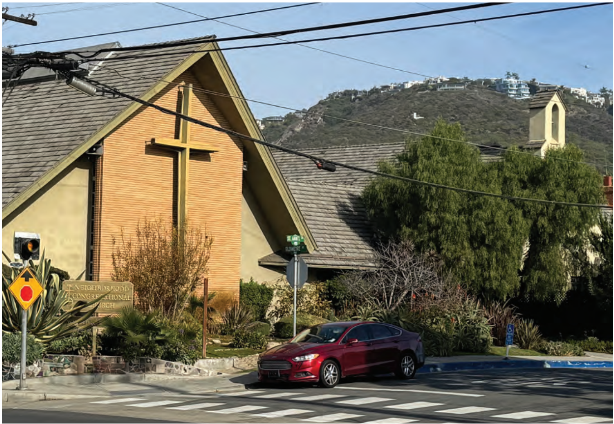
William Blurock Mid-Century Modern Church on left, Aubrey St. Clair Bridge (Parish) Hall, Tudor Revival, on right with bellcote
