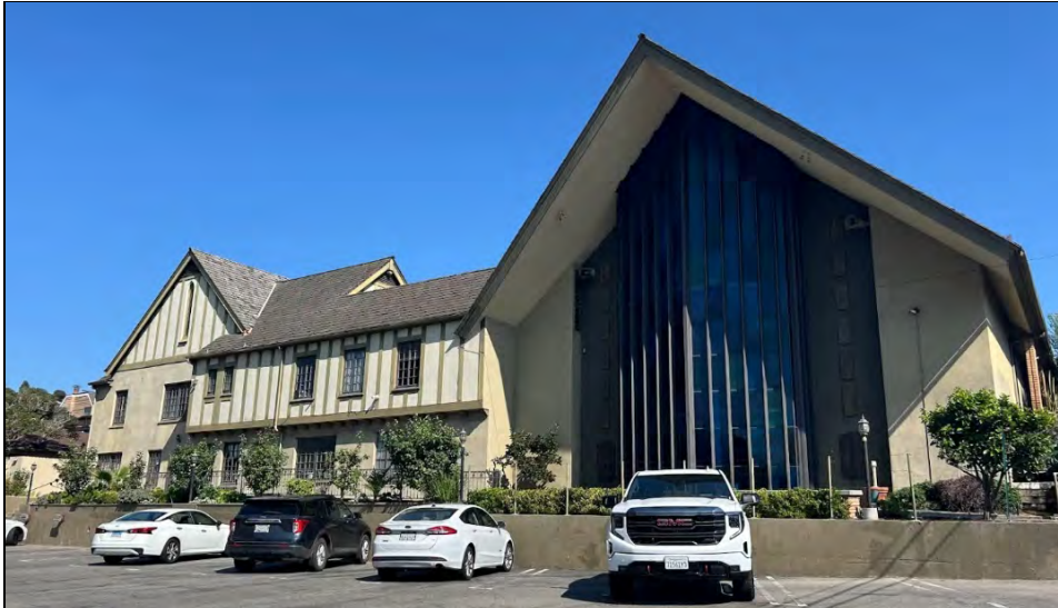
Photograph 4: Parish Hall at left, view southeast from parking lot. Note the half-timbered gable with lancet window the far left. It also features has a cantilevered, half-timbered main floor rear wall and complex intersecting roof forms. The asymmetrical Mid-Century Modern Church is at right side, its central, full-length windows jut outboard conjuring the bow of a ship. Photograph by Aaron Schrank for KCRW, permission pending. Not for publication.
