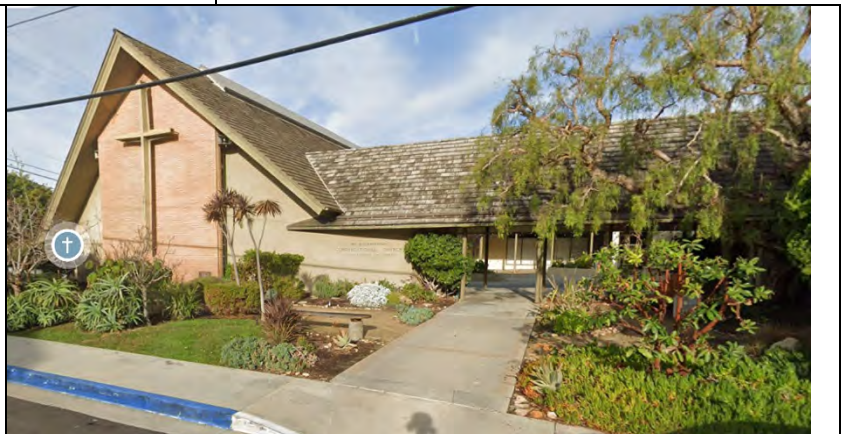
Photograph 6: Church, view northeast from Glenneyre. Note the soaring, asymmetric roof form and nearly full-length skylight at the ridge of the roof. The front roof plane extends on the left side to nearly meet finished grade. Narrow front and side windows are inset behind a "floating" brick wall. The simple shaped wood crucifix designed by a Blurock partner and was added in 1982. Note the seamless connection between the breezeway roof and the church roof. Google Maps September 2012.
