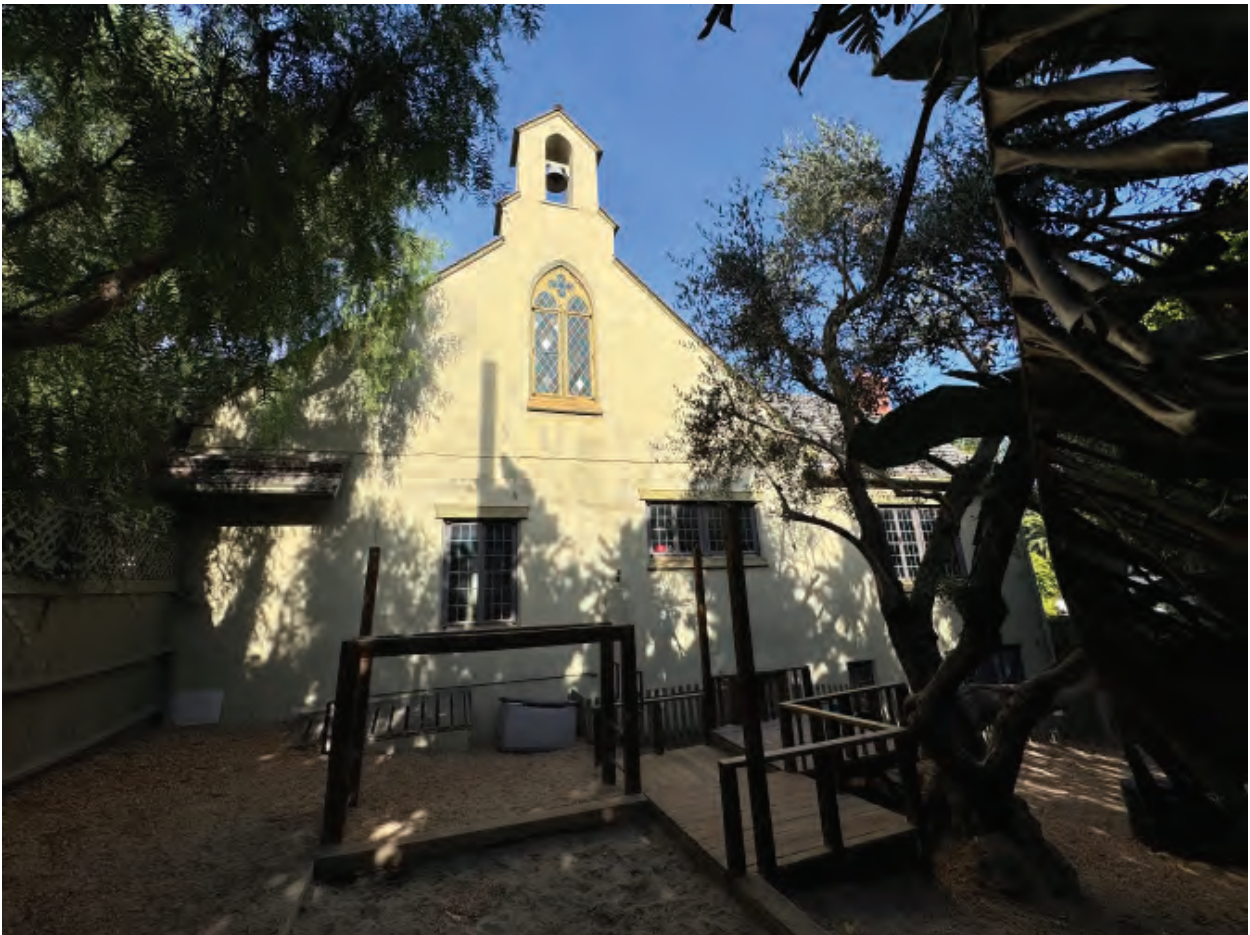
Bellcote of Bridge Hall
