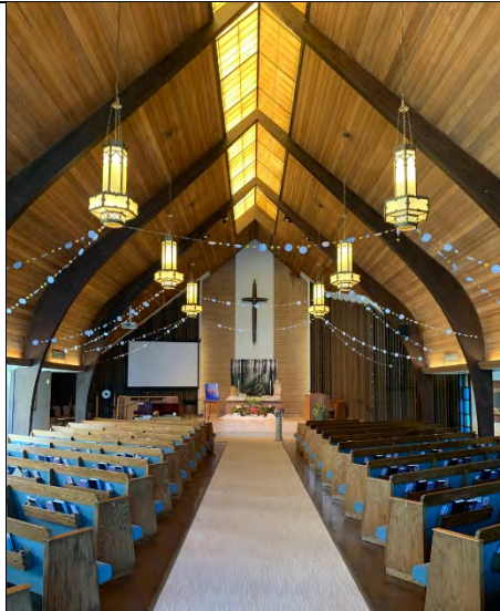
Photograph 8: Church sanctuary, view toward narthex. Note the darker glulam arches as well as the natural wood ceiling finish and the glass endwall. Photo by Hunter Fuentes, Historic Laguna. Not for publication.
