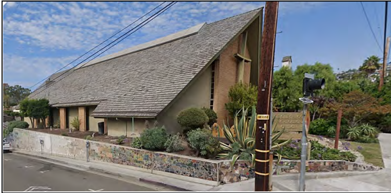
Photograph 5: Church, view northeast from Glenneyre. Note the soaring, asymmetrical roof form and nearly full-length skylight at the ridge of the roof. The front roof plane extends to nearly meet finished grade. The roof has rain diverters near the eaves to avoid the necessity for gutters, which would change the simplicity of the design. Narrow front and side windows are inset behind "floating" brick walls. Tiled retaining wall is in foreground. Google Maps September 2019.
