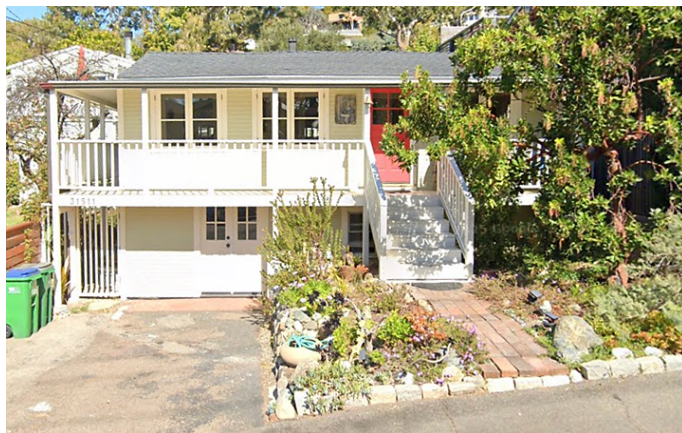
Figure 5. Relocated and remodeled James Shrewsbury house at 31511 Eagle Rock Way.
